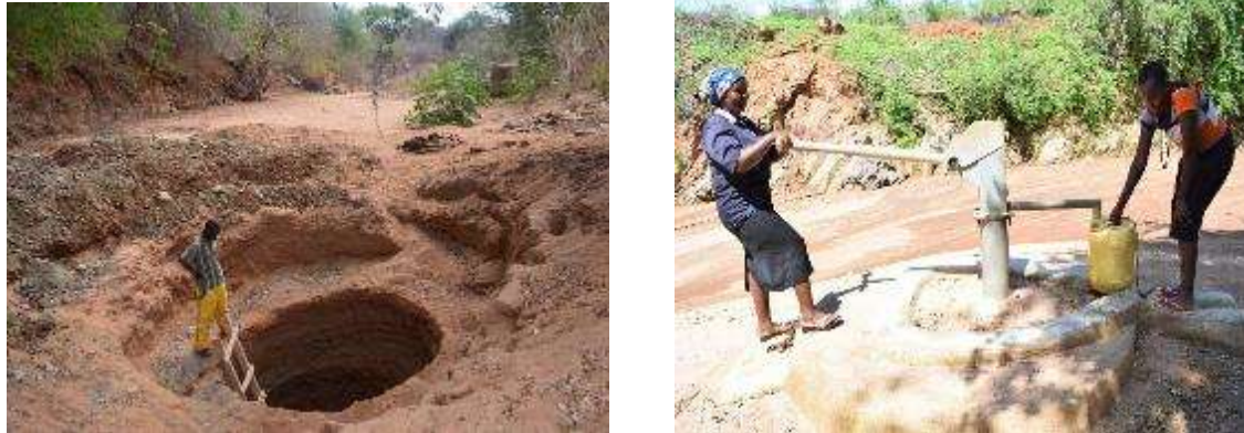
Figure 29: Shallow well works and a Borehole in use along a river in the Upper ACA (TWP, 2018)
