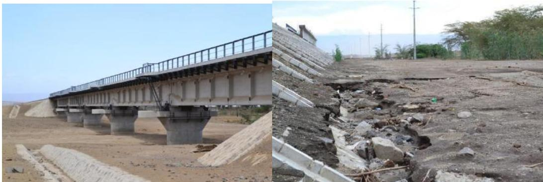
**Photograph 28&29:** SGR drainage structures interference with water flows and with impacts on the Suswa-Mai Mahiu Road
