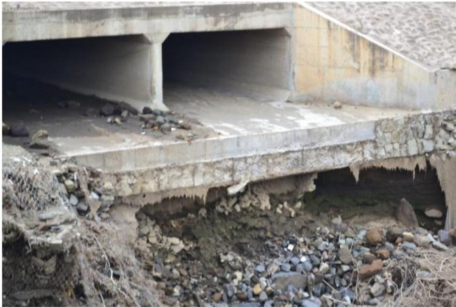
**Photograph 16:** Box culvert damaged by discharged floodwater
