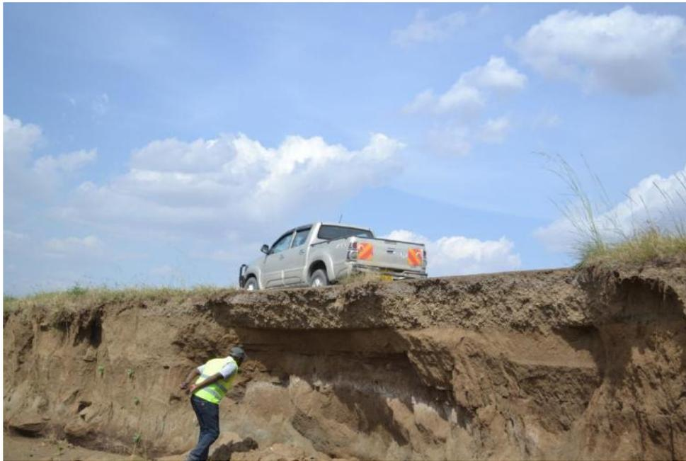
**Photograph 27:** Road foundation undermining by water in road parallel gully
