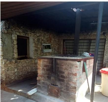
**Picture 2: The brick incinerator installed at the hospital**
