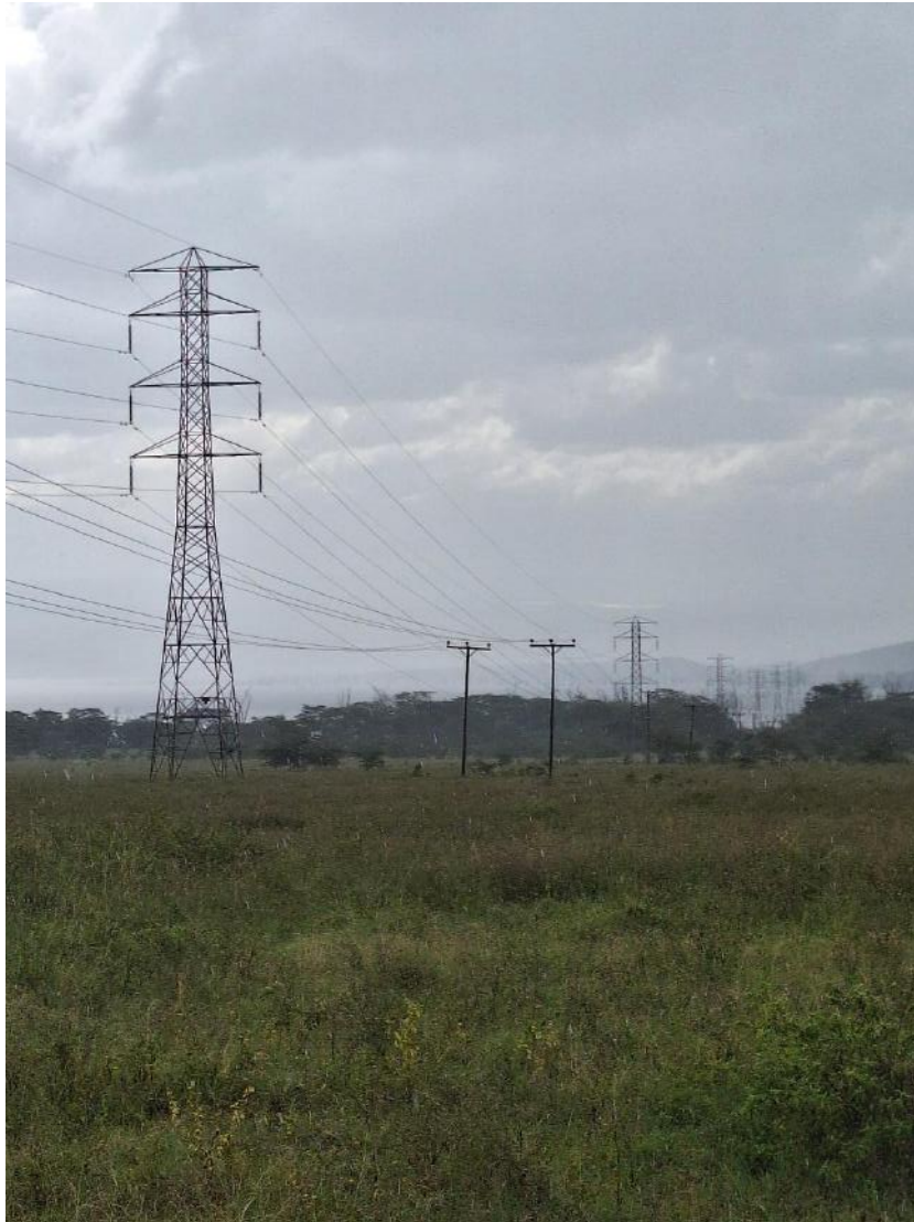
Photo showing a Section of the transmission line that shall be decommissioned and recovered.
