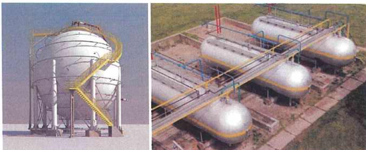
Plate 6: Typical spherical or horizontal and Horizontal Bullet LPG Storage Tanks
