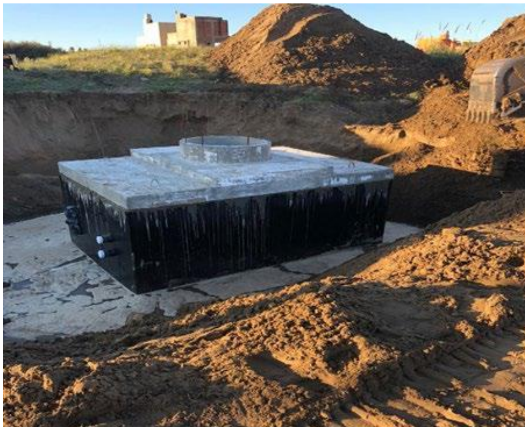
FIGURE 4-10 EXAMPLE OF A PREFABRICATED BEACH MANHOLE
