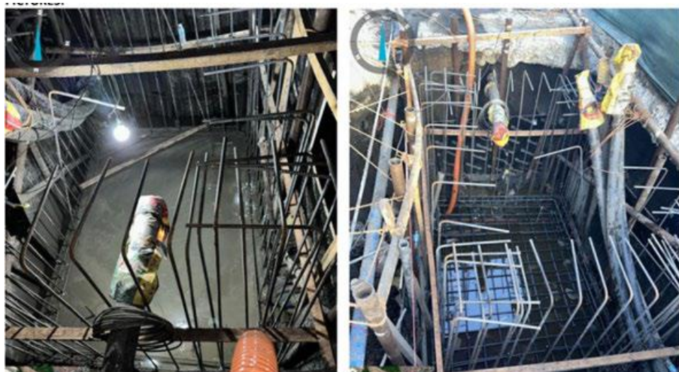
FIGURE 3-17 EXAMPLE OF BMH BEING CONSTRUCTED ON SITE WITH RE-INFORCEMENT BARS
