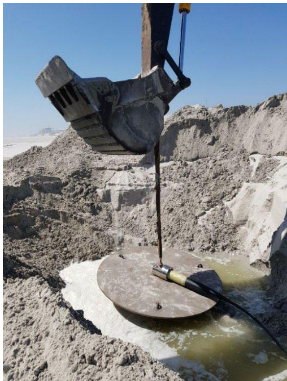
FIGURE 3-18 EXAMPLE OF BEACH PLATE INSTALLATION ON THE BEACH
