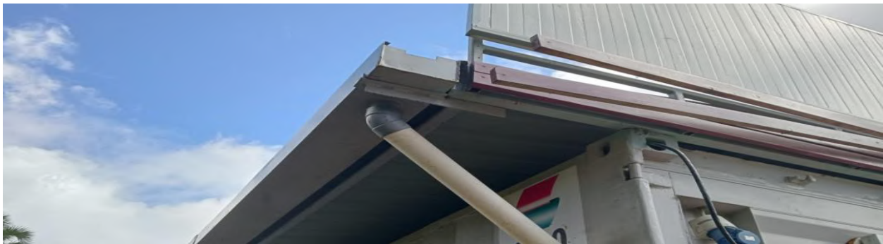
Figure 9-Roof Rain Water Catchment
