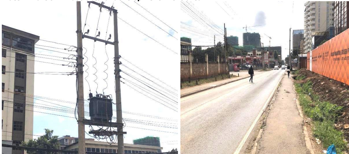
Plate 2: Part of infrastructural development in the area
