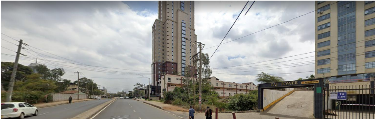
Tarmacked road, power line utilities serving the site area and environs
