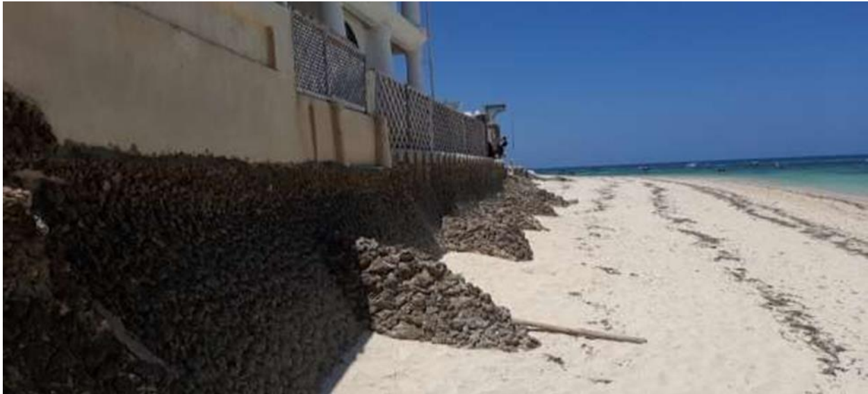
Plate 5: Typical Sea Wall
