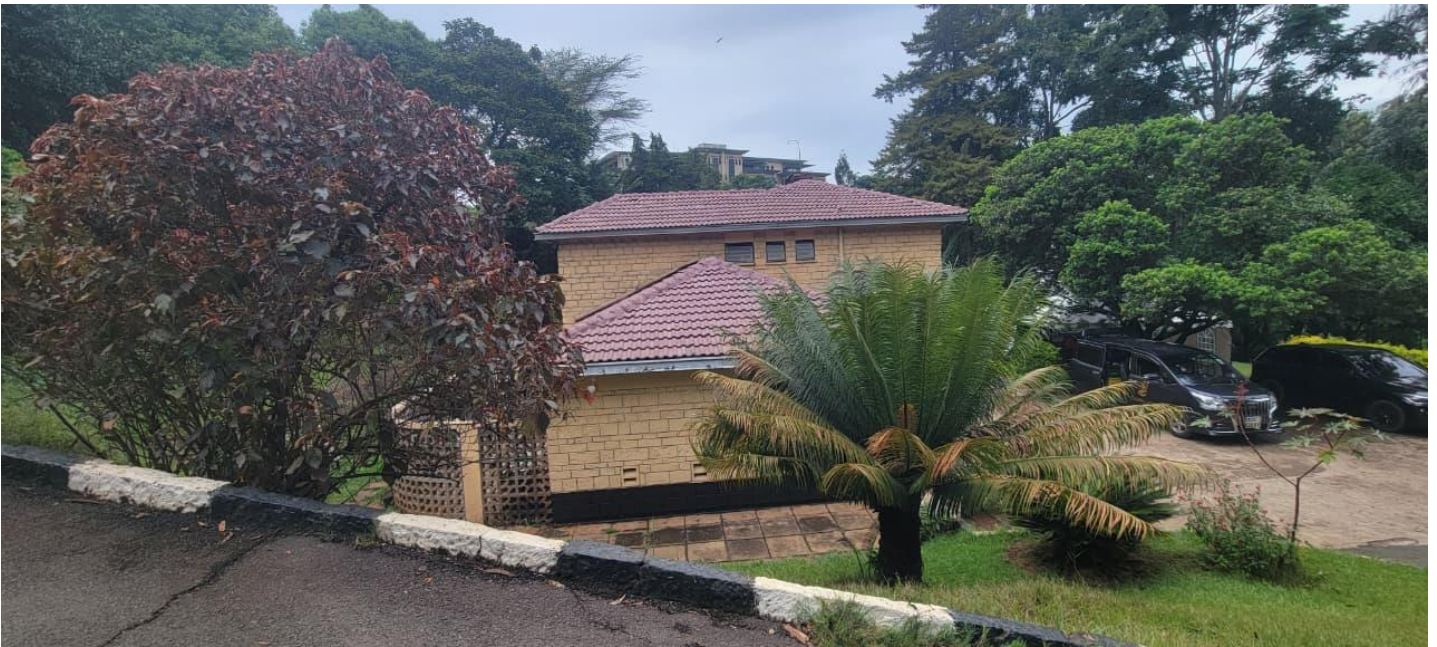
Figure 2: showing the current status of the project site.
