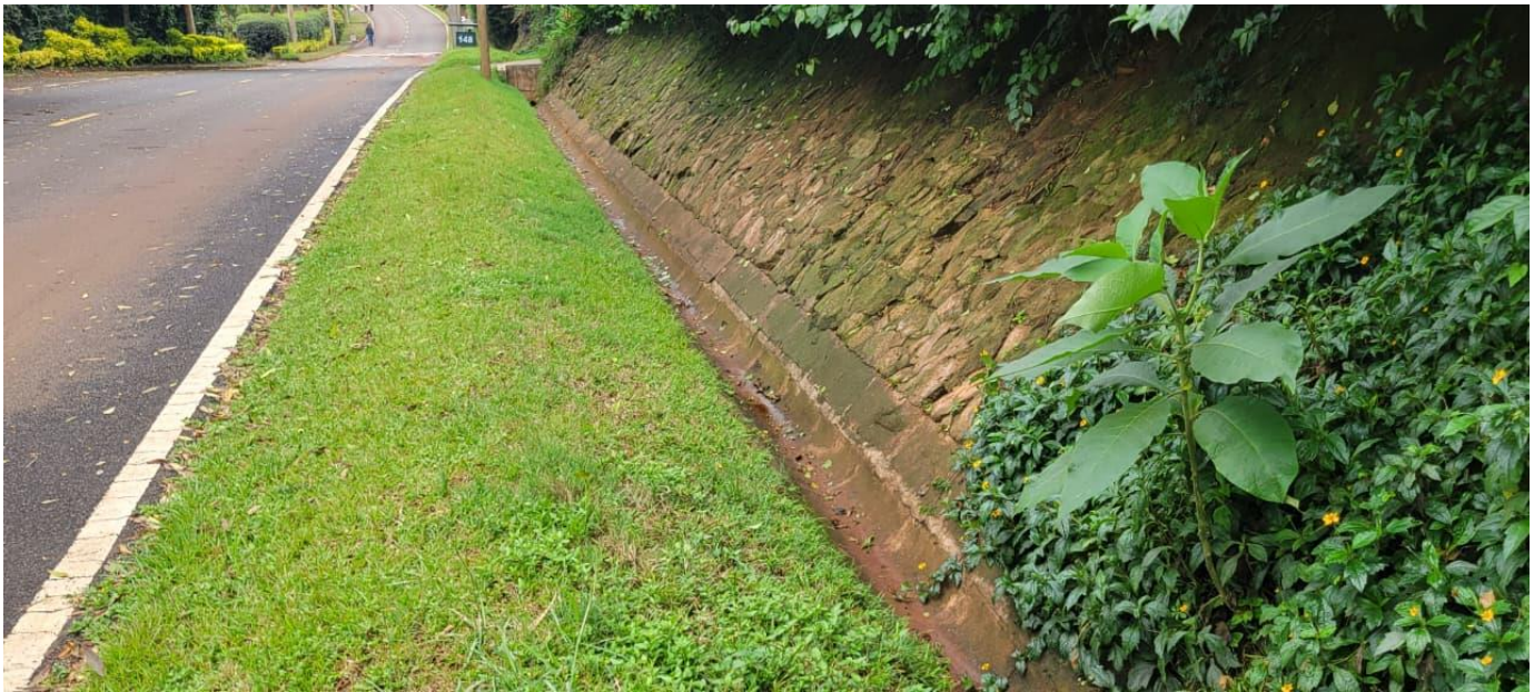
Figure 5: showing stormwater drainage channel along UN crescent road.
