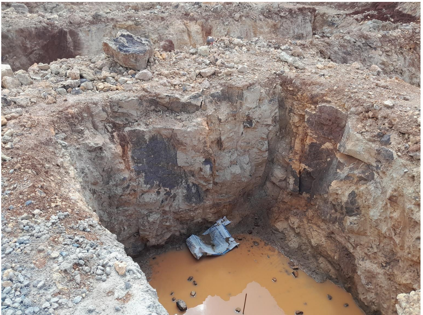
Plate 1: A test pit drilled during geotechnical investigations
