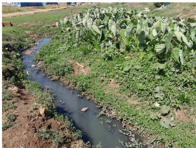
Plate 14: Raw sewage within the project neighborhood
