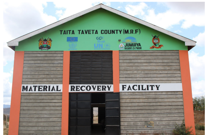
A Material Recovery Facility (MRF) at Mwatate, Taita Taveta County
