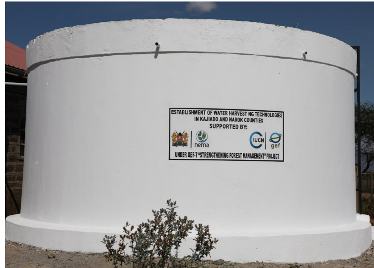
The masonry 10,000L water tank constructed at Olodungoro Primary School through GEF-7 project.
