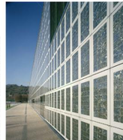
SOLAR PV SKIN ON BUILDING FACADE
