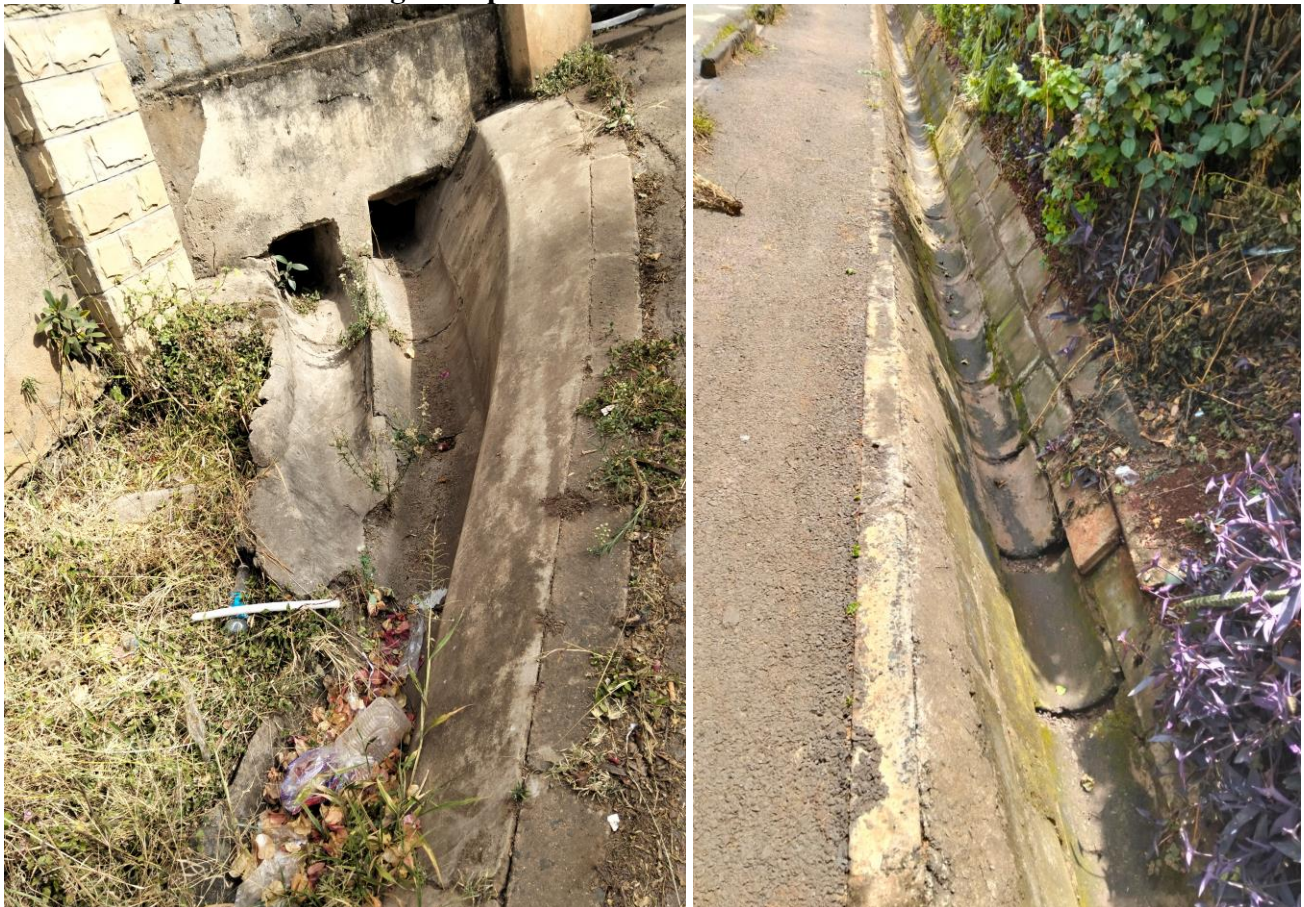
Plate 2. 6: Open Drains along Laikipia Road
