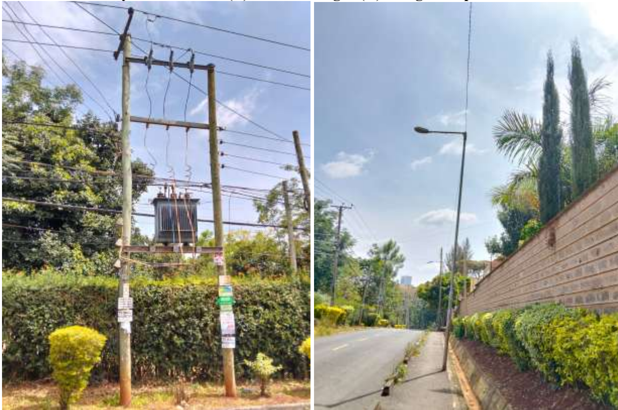
Plate 4: Electricity Transformer (L) and Streetlight (R) along Laikipia Road
