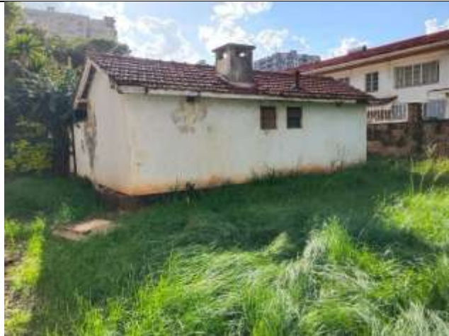
Image 4; View of the proposed site (building at the rear side)
