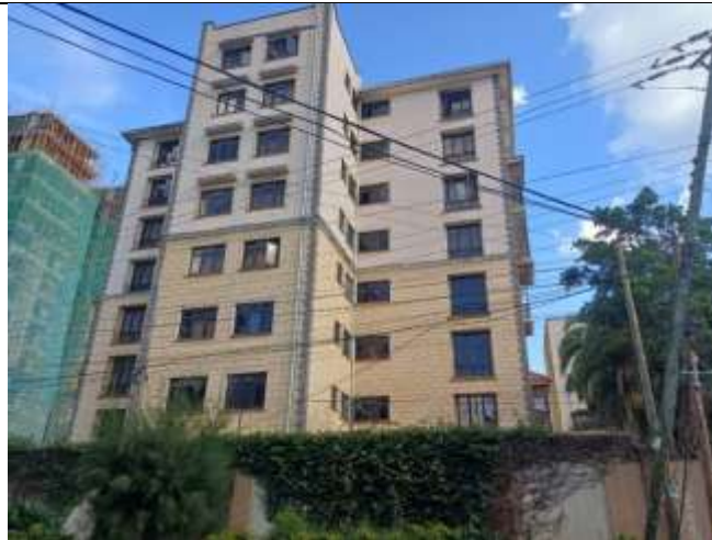
Image 8: View of the opposite building along Kilimani road
