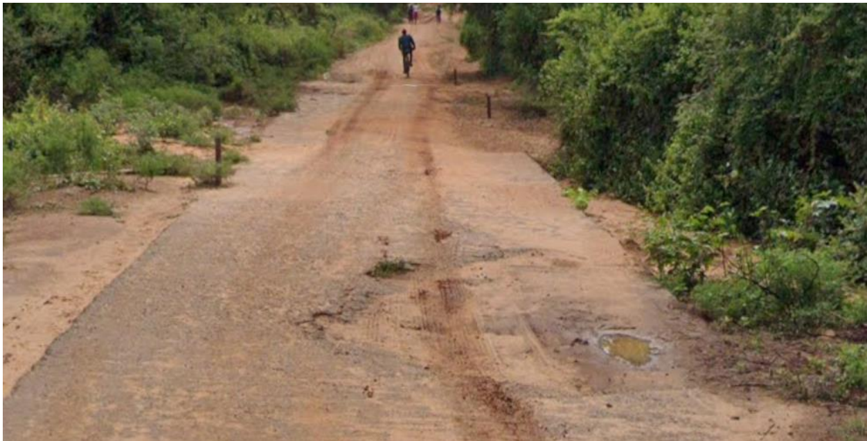
Plate 6: Access Road (Ikutha-Nguuni Road)
