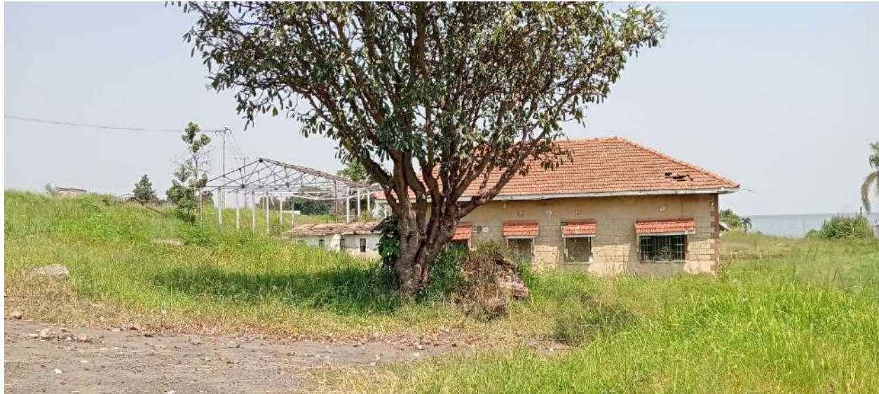
Figure 19: Structures on adjacent land (Proposed KPA Passenger terminus site) to the proposed project site (Source: Site Visit, June 2024)
