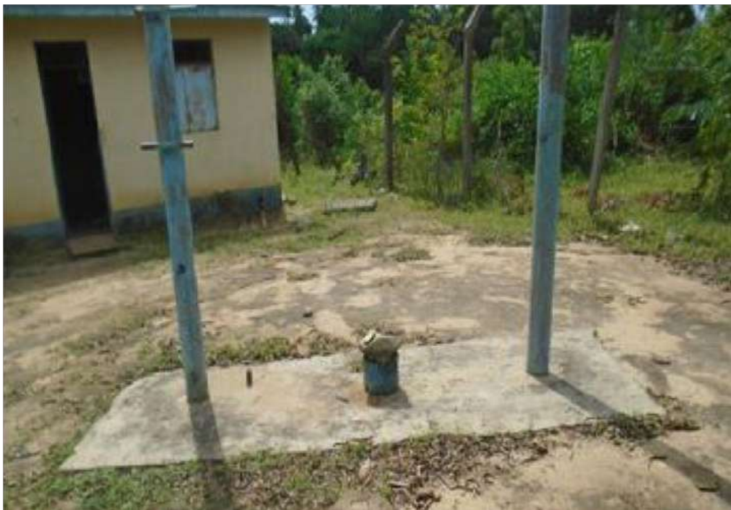
Figure 15: Borehole A one of the main sources in Tiwi Well field to Kaya bombo reservoir
