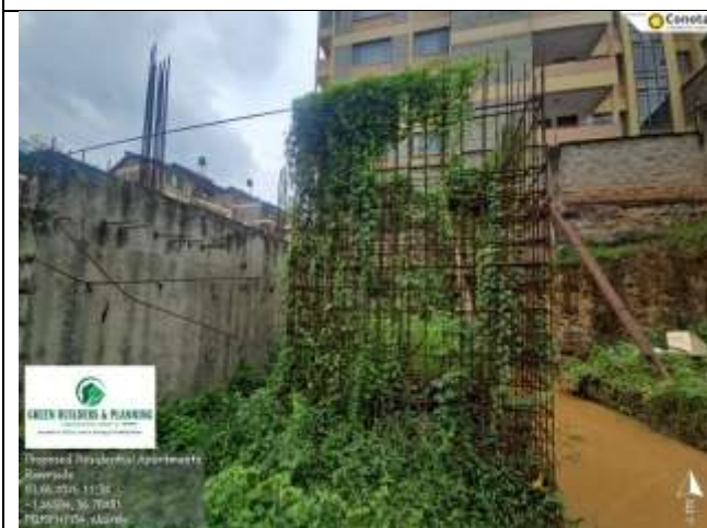
Image 4 and Image 5; Existing unfinished foundation on the project site set for demolition to allow for redevelopment of the proposed residential apartment building.
