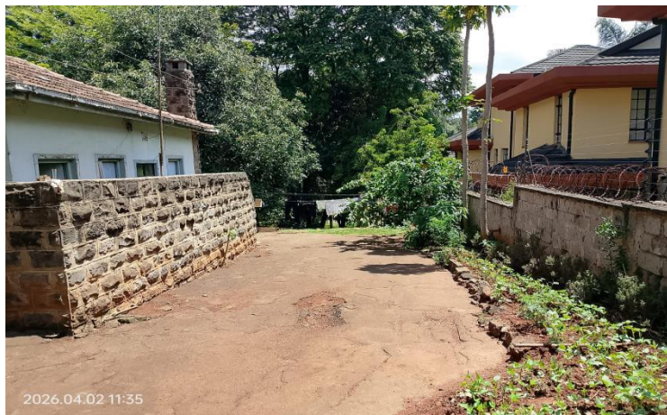
The Project Site
