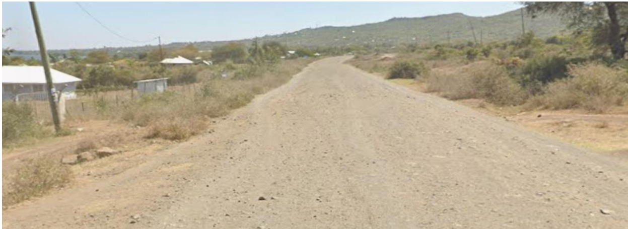
Plate 7: (C19) Mbita-Sindo Access Road
