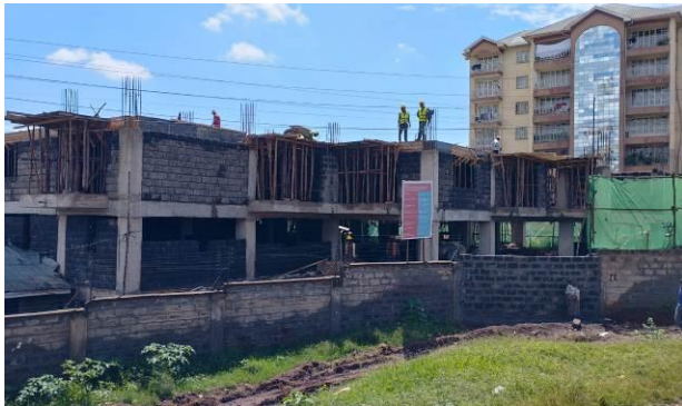
Plate 3: A residential under construction near Waterfront apartments
