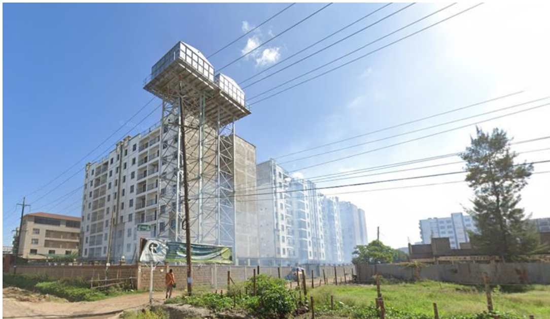
Figure 4 Photograph showing ongoing development within the neighborhood (Source Google Street 2024)
