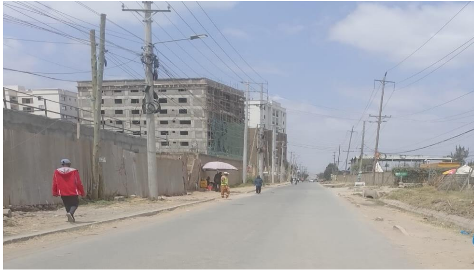
Figure 6 A photograph showing the current status of the road and the street lighting infrastructure
