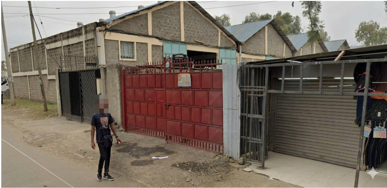
Plate 13: Godowns Along Workshop Road
