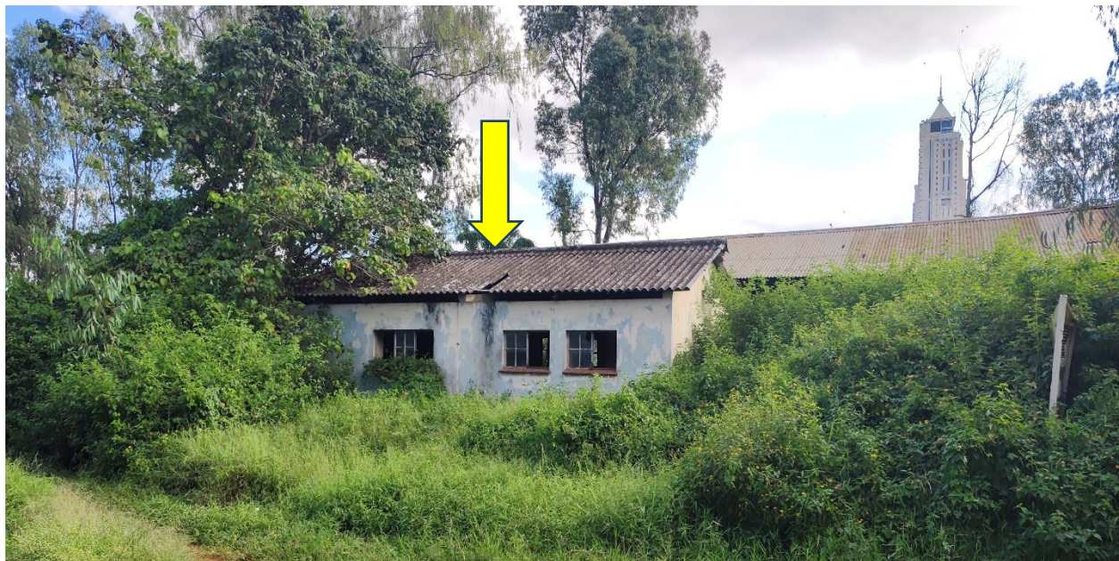
Plate 30: Site Structure with Asbestos Containing Material
