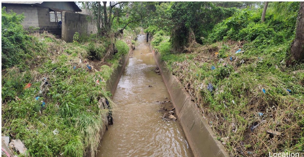
Plate 2: Drainage System (Tributary of Ngong River Canal) along the Project Boundary
