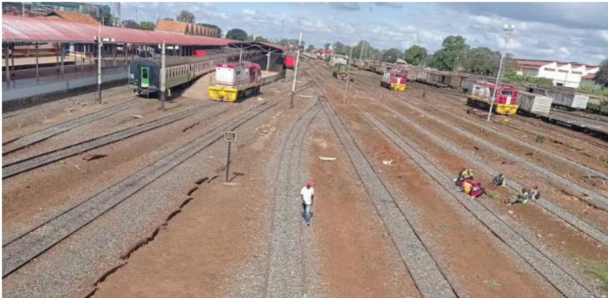
Plate 17: Active Railway Line (Source: Kenya Railway)
