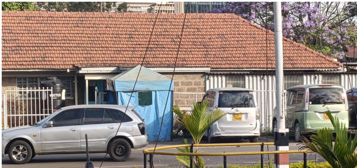
Plate 16: Loco Health Centre Near Over Pass Bridge-Workshop Road
