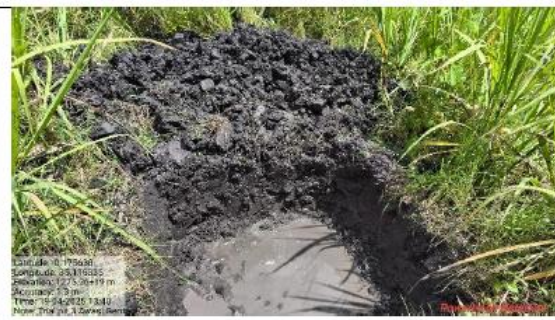
Trial Pit 3 logged with surface water infiltration
