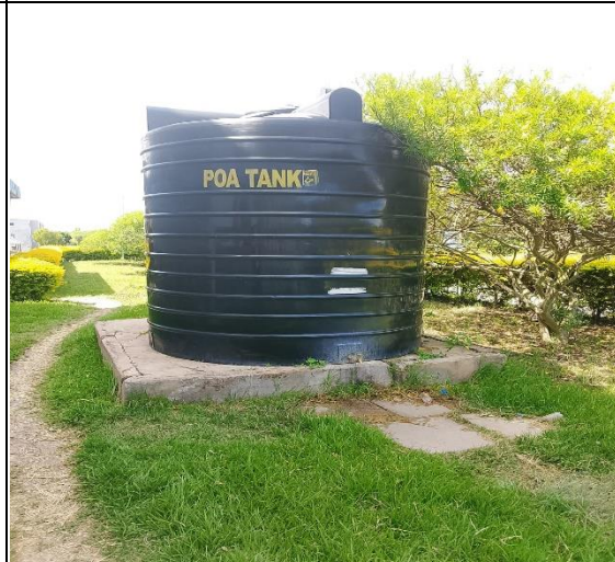
Existing storage tanks
