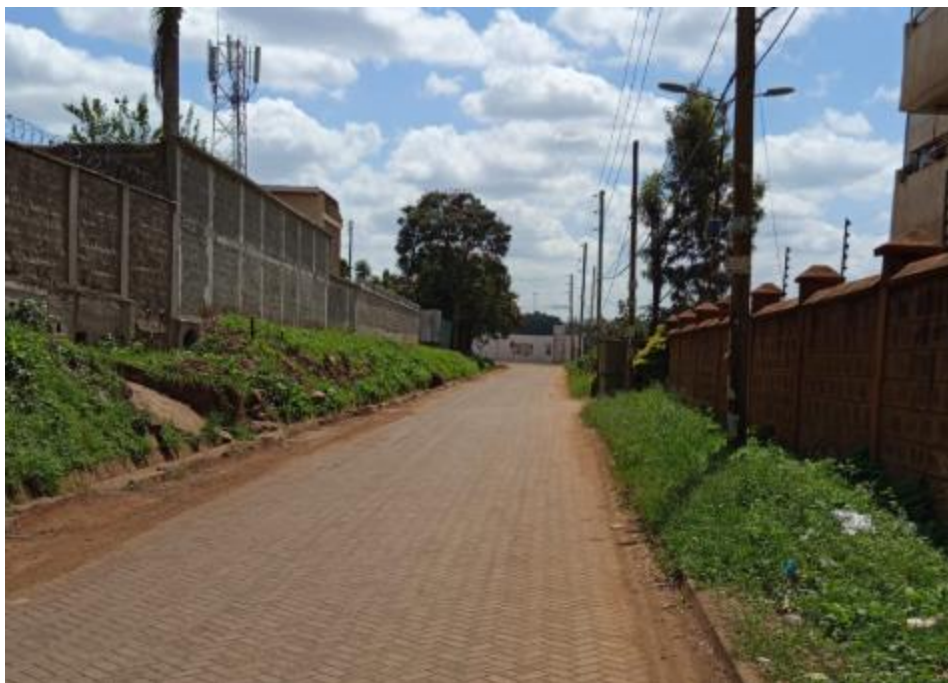
Plate 2-5: Access Road to the site
