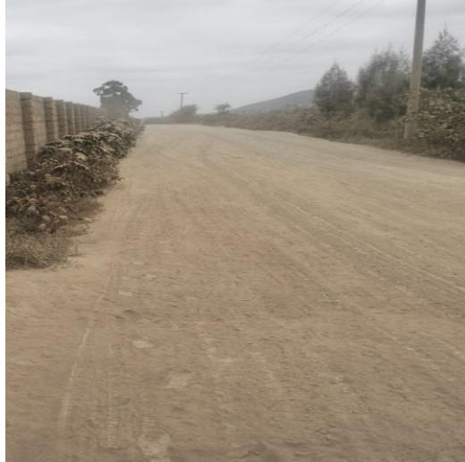
Three phase powerlines within project vicinity
